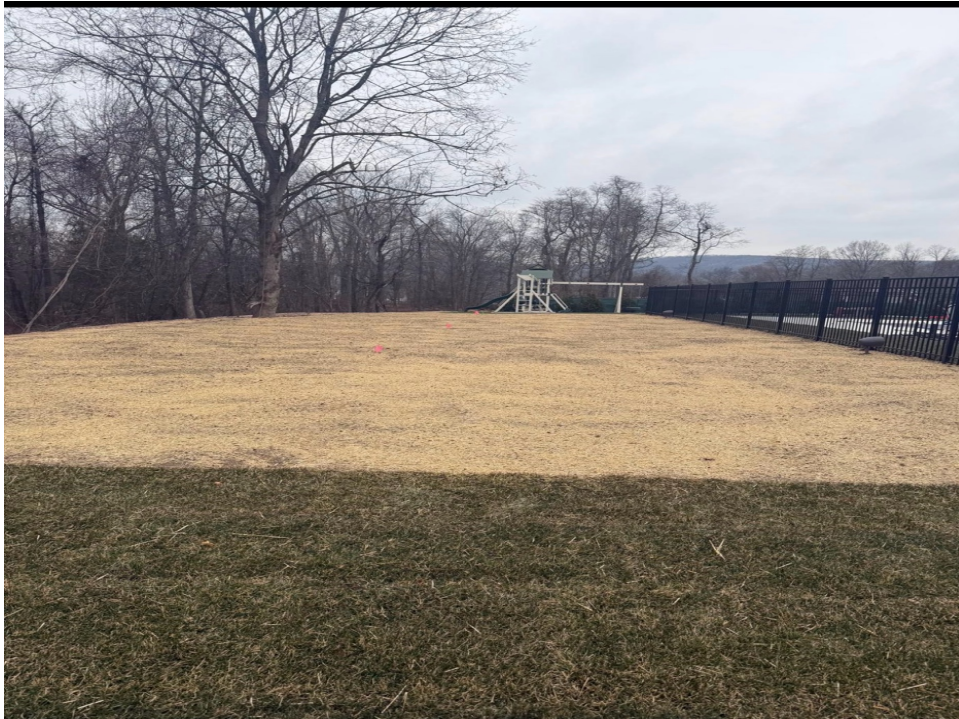
Photo 6: Backyard showing fill work creating level play area
