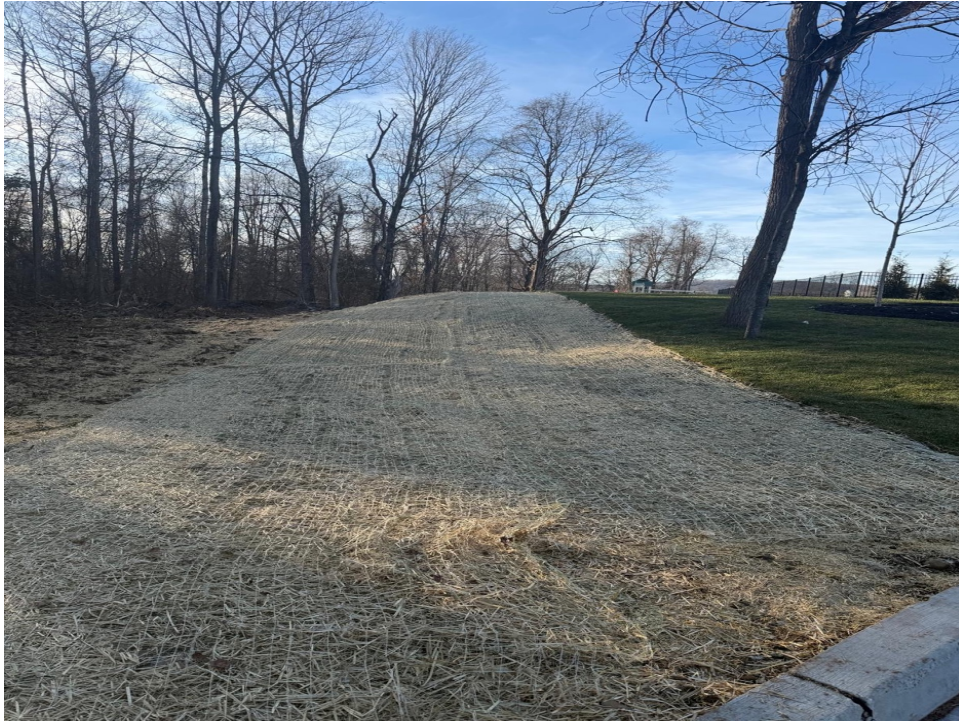
Photo 1: Graded area with erosion control matting and established lawn
