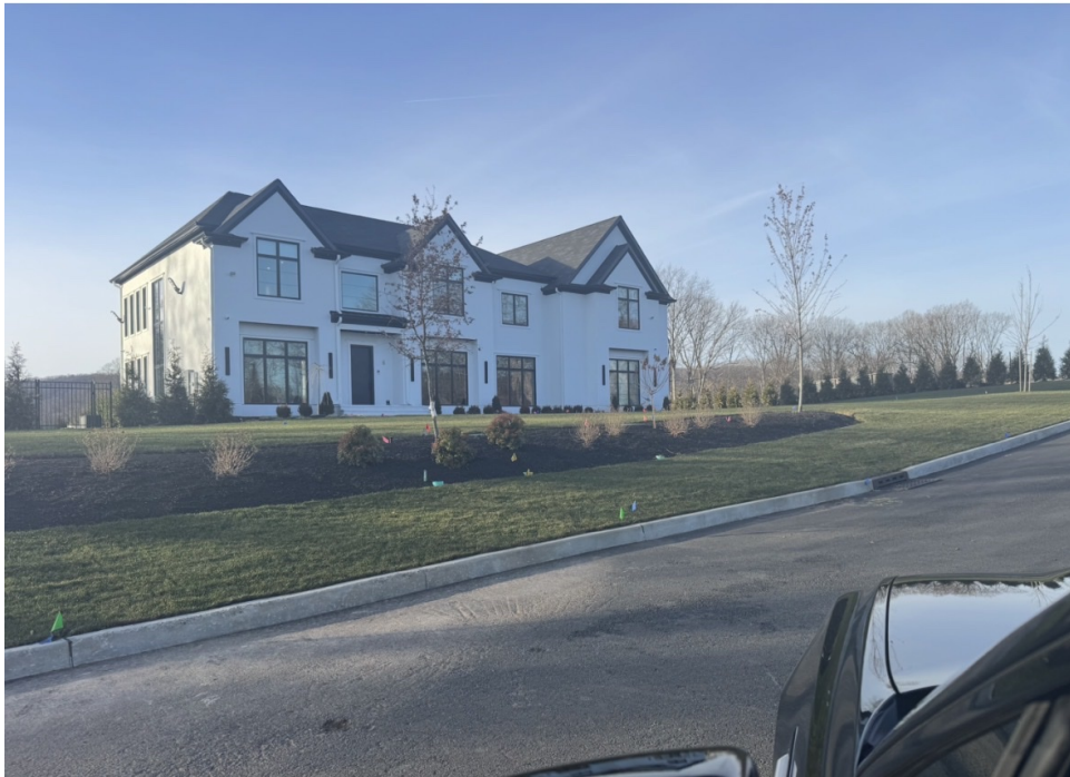
Photo 4: Front view of property with completed landscaping
