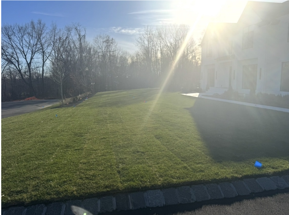
Photo 3: Side yard showing graded and seeded area
