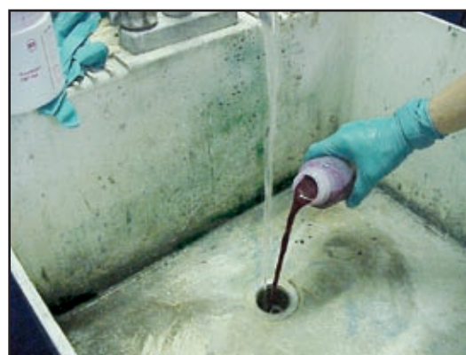
Figure 63: Dye Testing Plumbing (NEIWPC, 2003)
