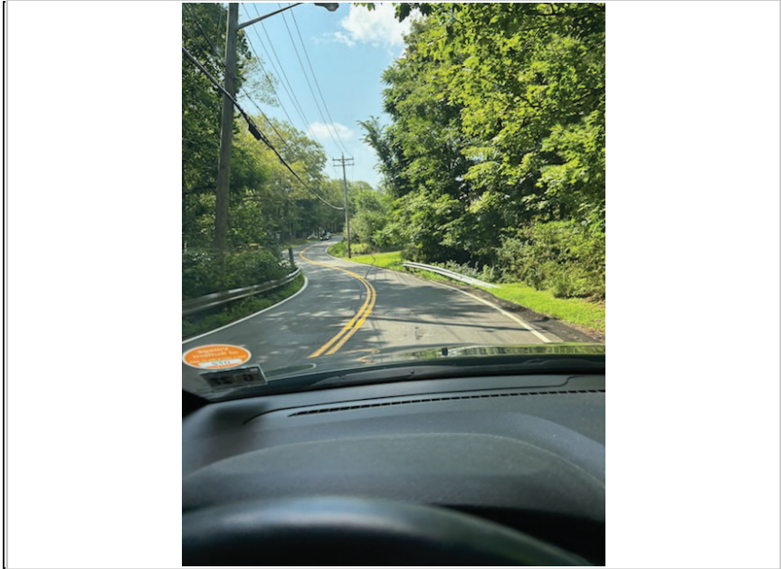
View for vehicles traveling southbound on McNamara Road prior to horizontal curve.
