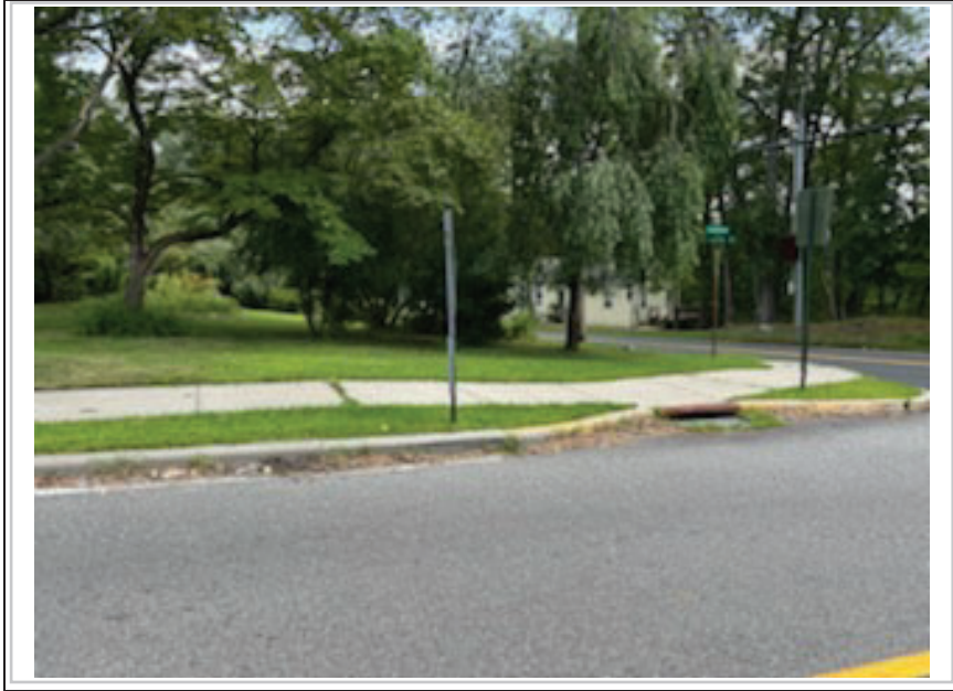
Sight distance for vehicles on East Willow Tree Road looking north, stopped at stop sign.
